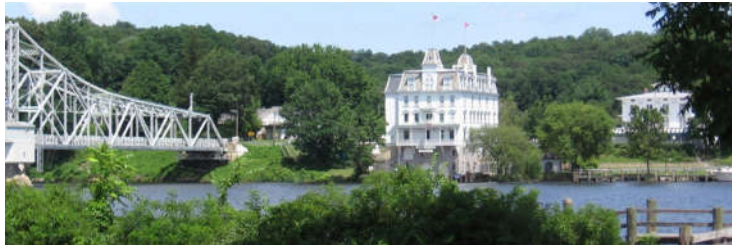
Goodspeed Opera House on the Connecticut River
